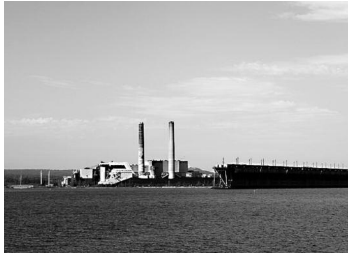
We Energies Presque Isle Power Plant in Marquette Michigan.
